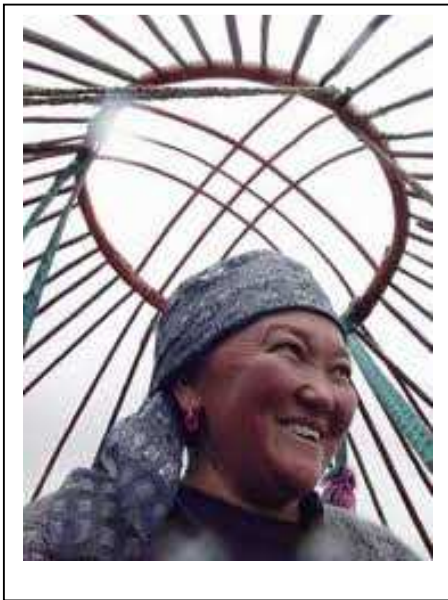
A view of the tunduk from inside the boz ui before the sheepskin outer covering is added.
